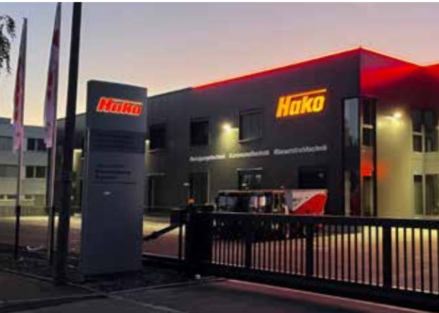
Franken subsidiary, new build to the KfW40 standard
